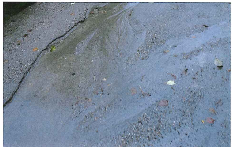
CK2002 Deck sediment from left
