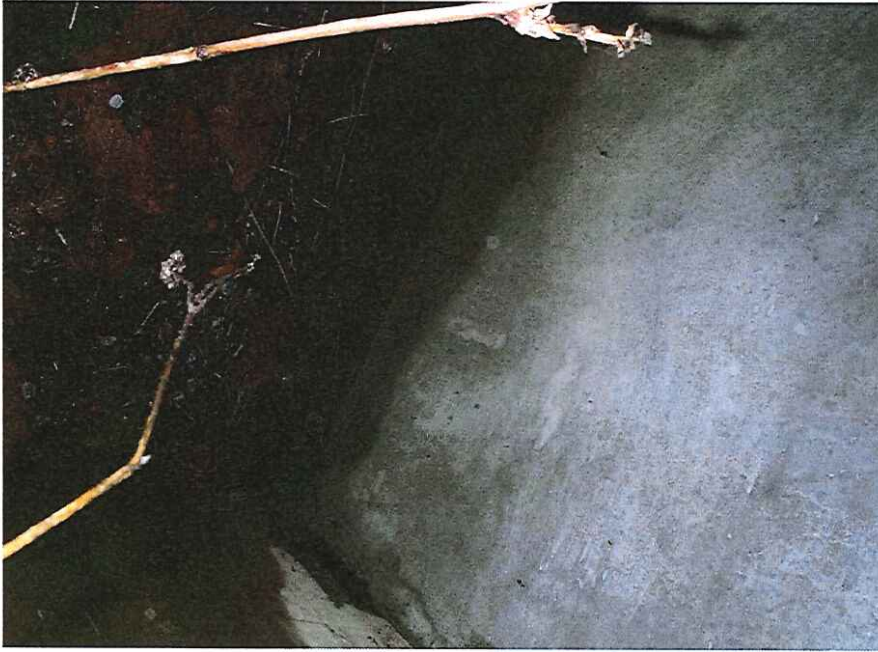
CK2002 Left Abutment bearing
