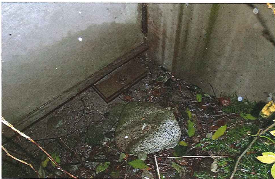
CK2002 Right Abutment bearing
