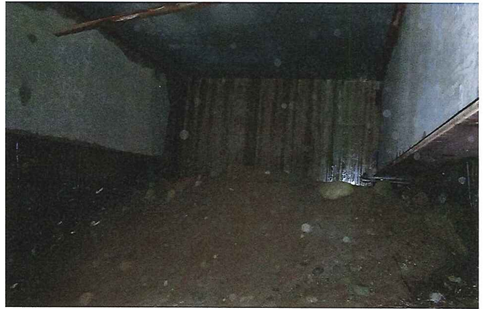
CK2002 Right Abutment
